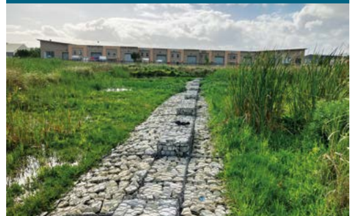
Construction of a gabion weir across the Asanda wetland to spread flows.
