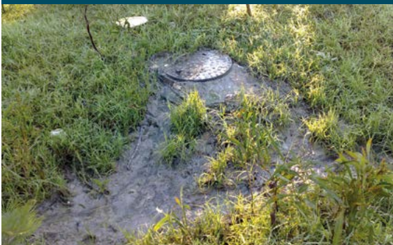
Overflowing sewer manhole, leading to the Sir Lowry's Pass River.
